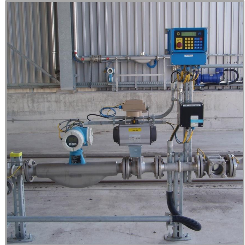
Truck loading system bio fuels with the Endress+Hauser mass flow meter Promass 84F
